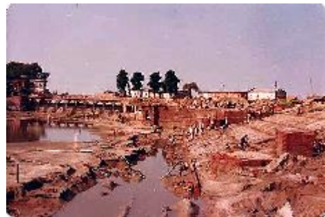
PEDESTRIAN BRIDGE ACROSS WATER CHANNEL AT AYODHYA
