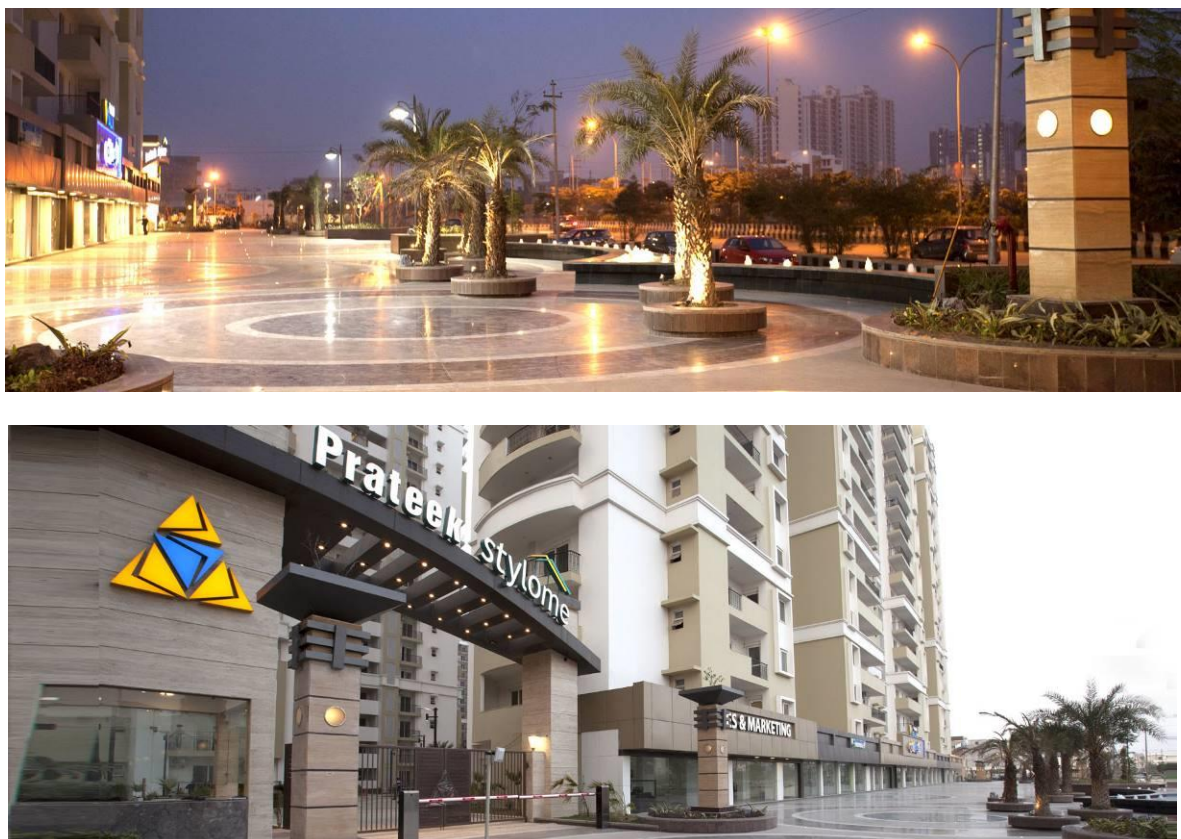
7.28 Prateek Stylome housing at Noida, UP in 7.44 acres of land for Prateek Realtors India (P) Ltd. designed by Deepak Mehta & Associates, New Delhi.
