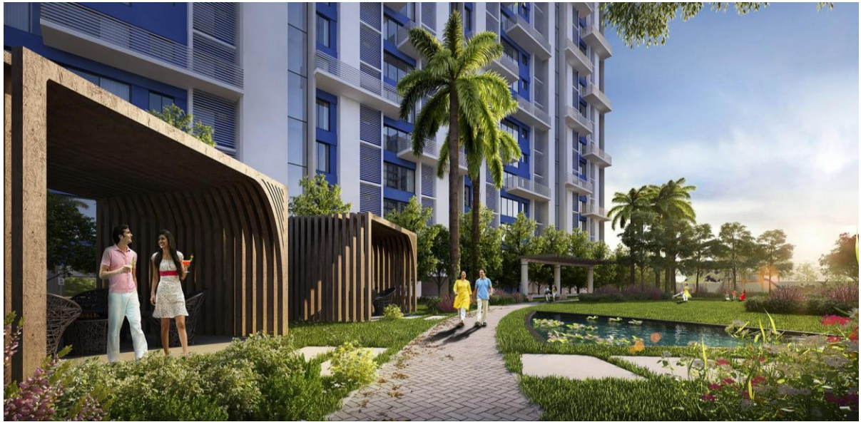
7.117 Sugam Diamond Morya Housing at Kolkata in 5.25 acres of land for M/s Sugam Diamond Abasan LLP, Kolkata designed by M/s Innate, Kolkata– ongoing project.
